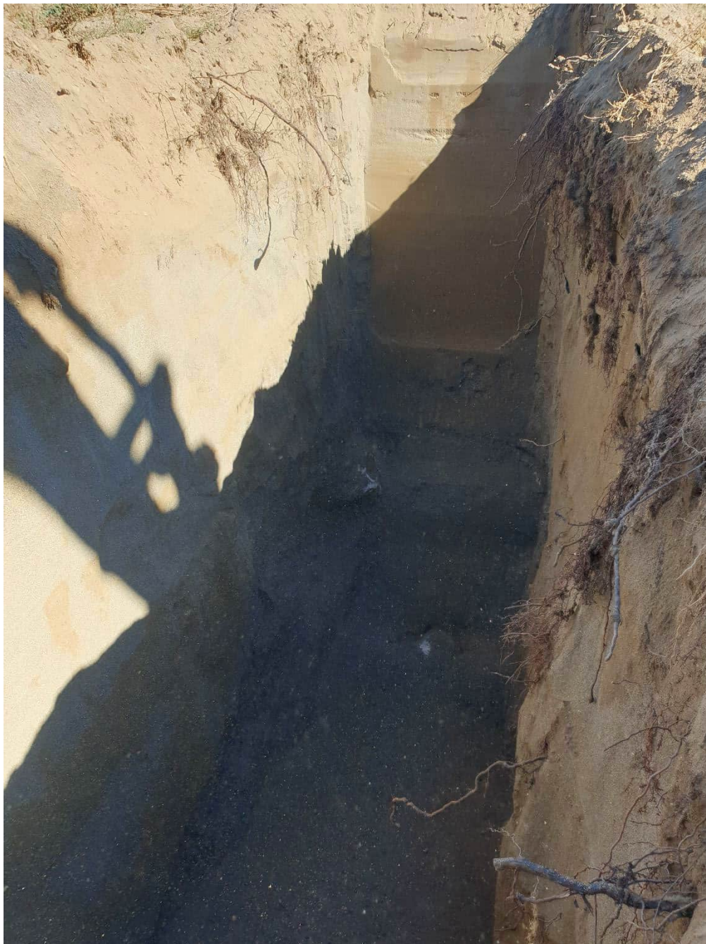
TP07 – TEST PIT EXCAVATION
