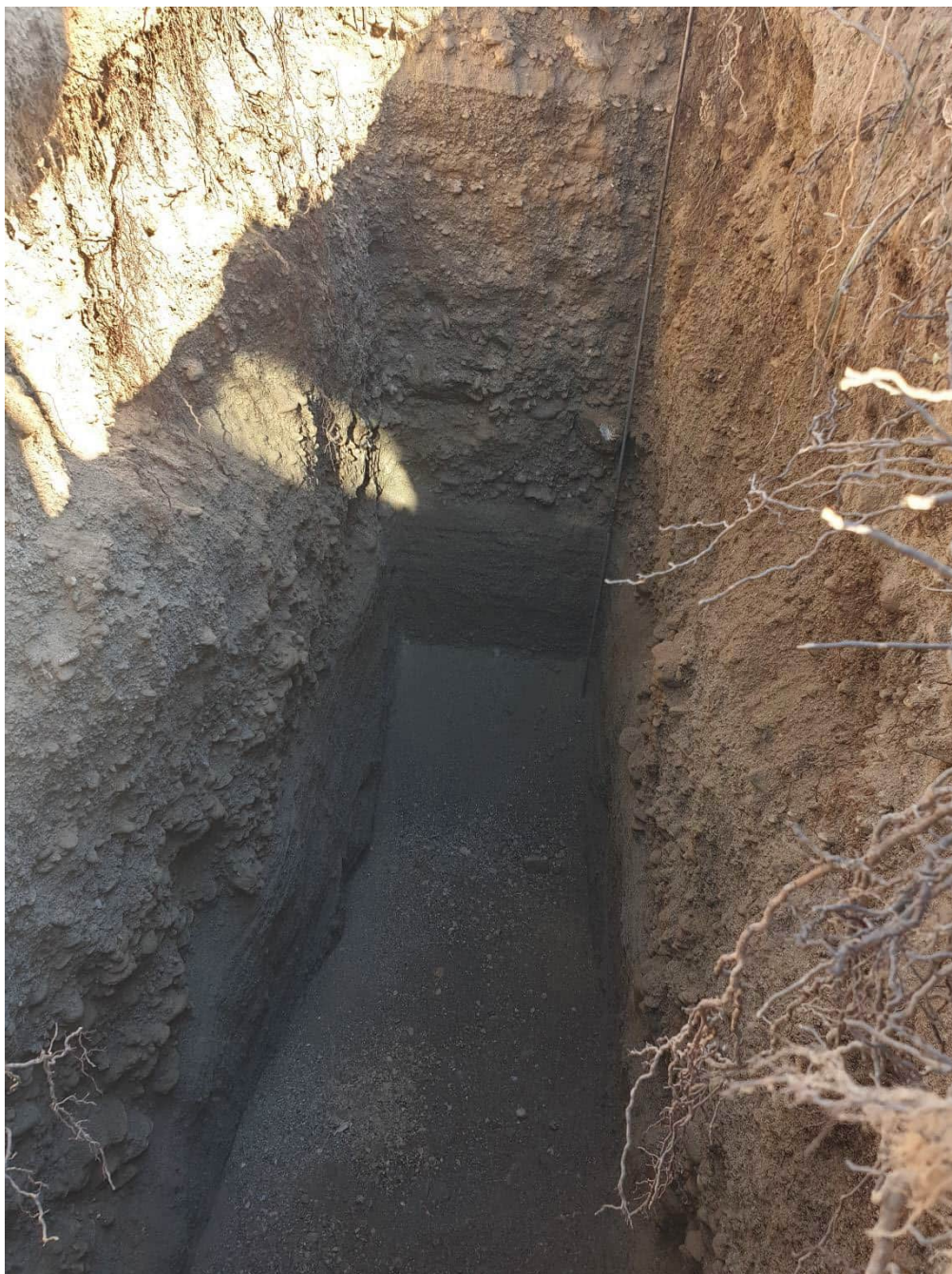
TP05 – TEST PIT EXCAVATION
