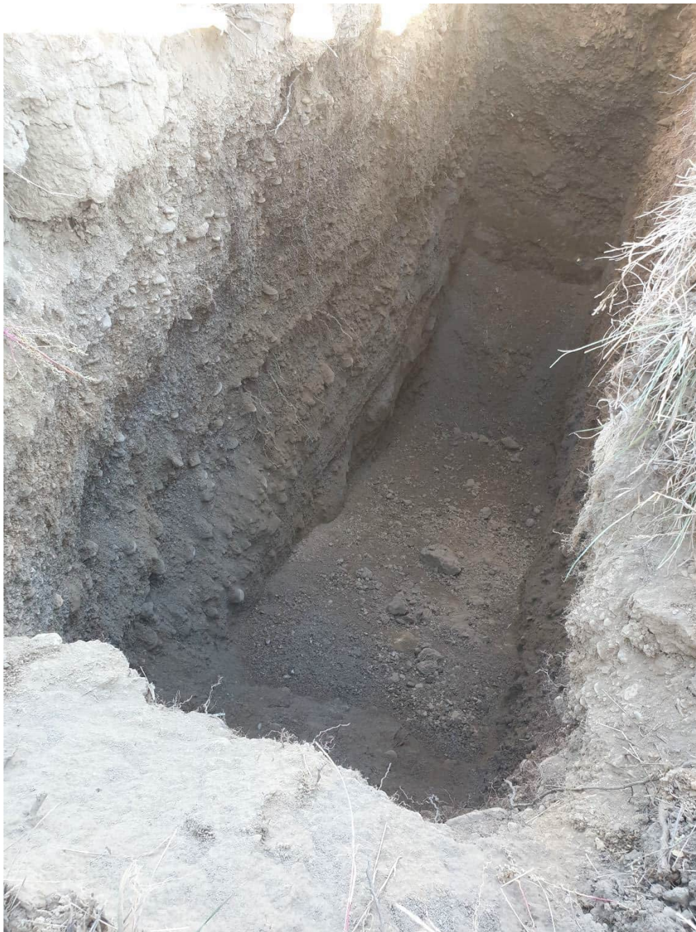
TP02 – TEST PIT EXCAVATION
